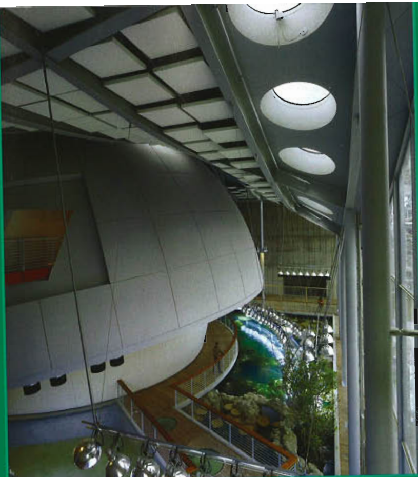
The exterior of the Morrison Planetarium.
