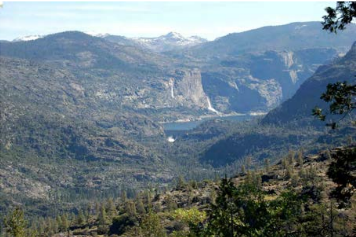
Figure 56. Hetch Hetchy Valley, O'Shaughnessy Dam and Hetch Hetchy Reservoir (SFPUC).
