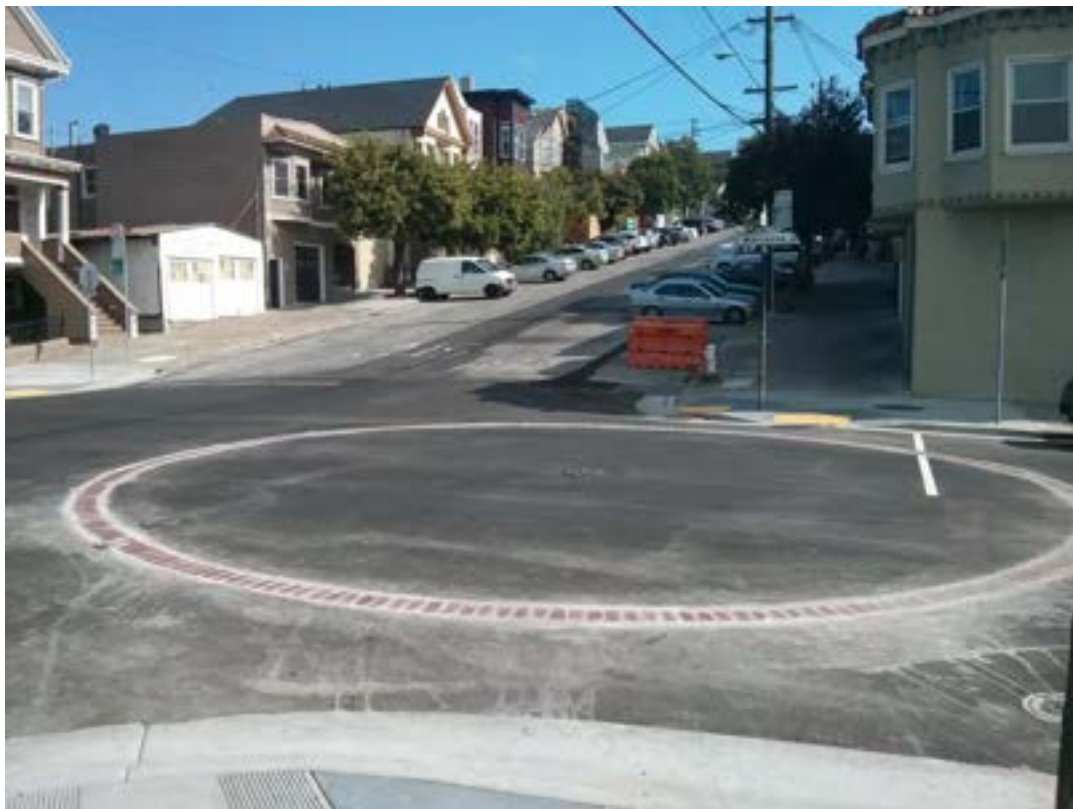
Figure 58. Typical emergency water supply cistern at intersection of Mariposa Street and Missouri Street (Mark Hogan).
