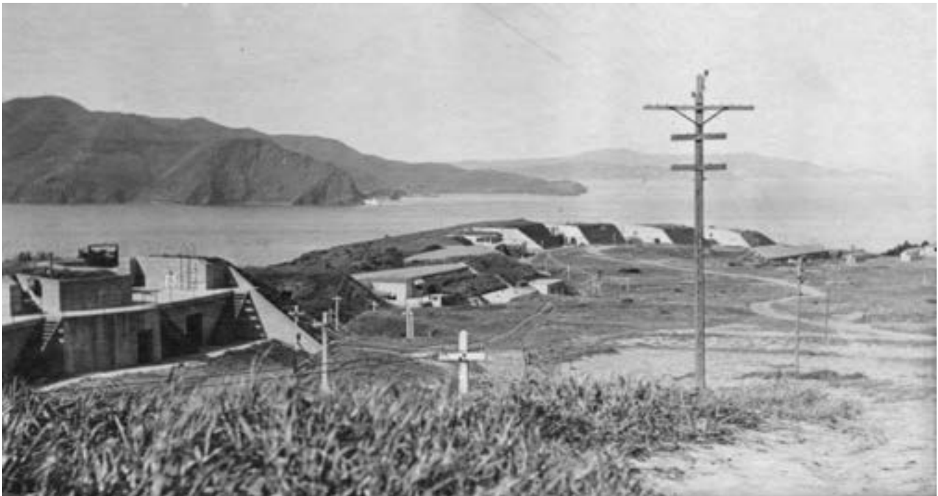
Figure 70. Endicott batteries at Fort Scott along the former location of West Battery. L to R: Batteries Boutelle, Marcus Miller, Cranston, and Lancaster (John A. Martini Collection).
