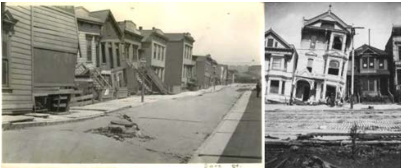
Figure 50. Liquefaction-related damage in San Francisco due to the 1906 earthquake. Photograph on left shows Dore Street (from Bancroft Library) and photograph on right shows an area near Howard & 17 th Streets (G.K. Gilbert, USGS photo).
