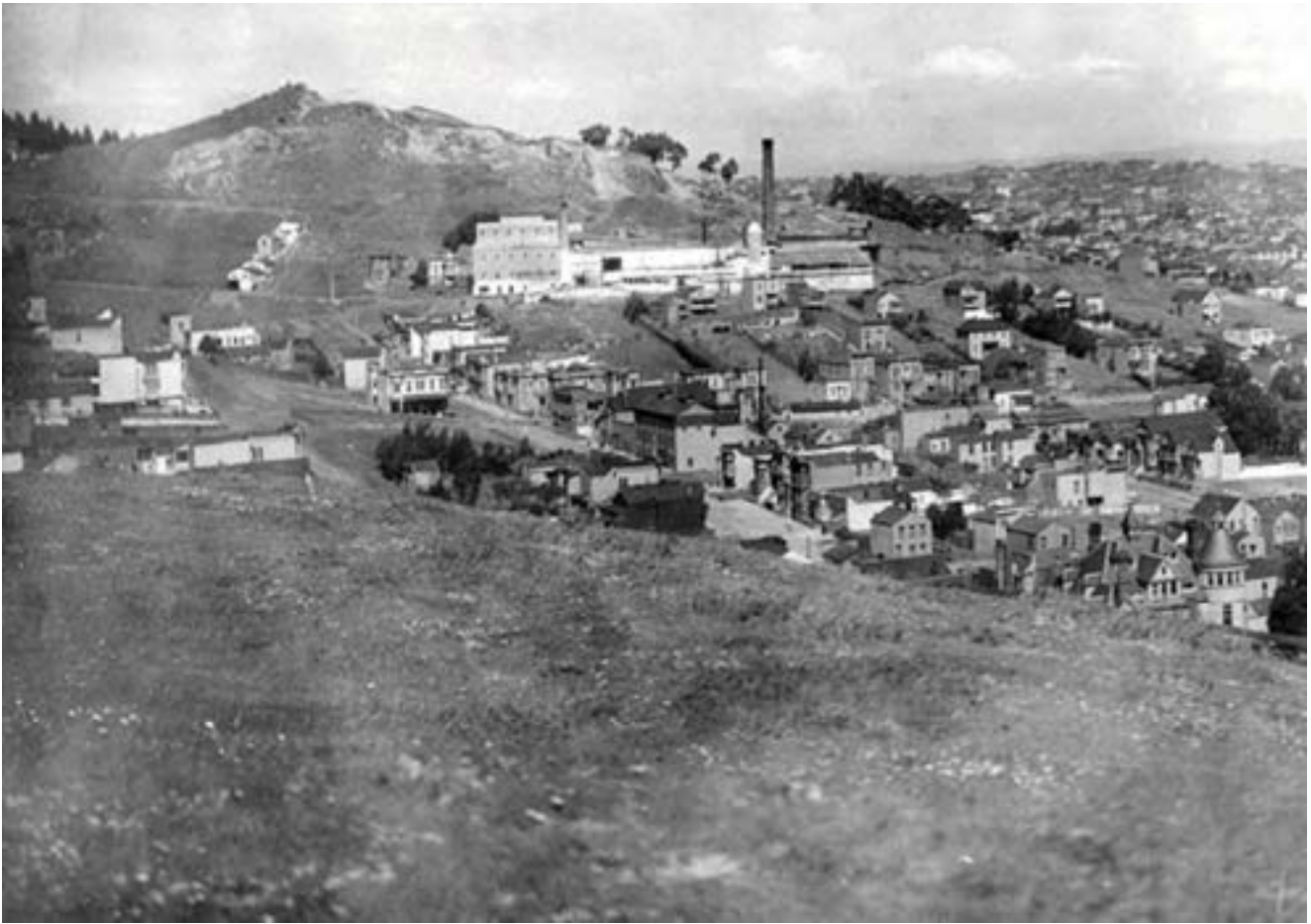
Figure 15. The Gray Brothers Quarry and Brick Factory in Corona Heights, 1888 (FoundSF.org).
