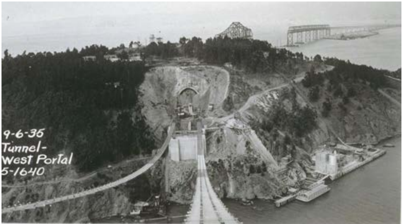
Figure 79. West Portal of the Yerba Buena Tunnel during construction of the San Francisco–Oakland Bay Bridge, as seen from the first tower of the western span; notice eastern span in background (Bancroft Library Collection).
