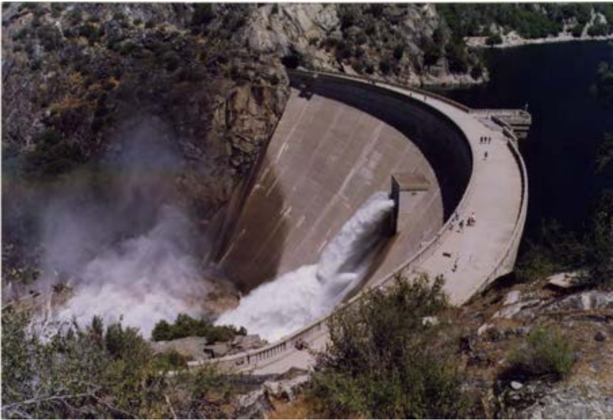
Figure 55. O'Shaughnessy Dam and Hetch Hetchy Reservoir (SFPUC).
