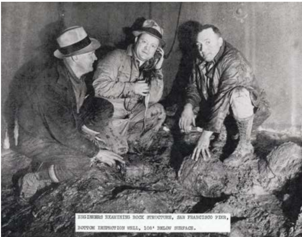
Figure 76. Engineer team at the bottom of the south pier excavation; note the stylish hard hats of the time (Willis, 1934). From Golden Gate Bridge and Highway District, Investigation of criticism of foundation by Bailey Willis, November 27, 1934.
