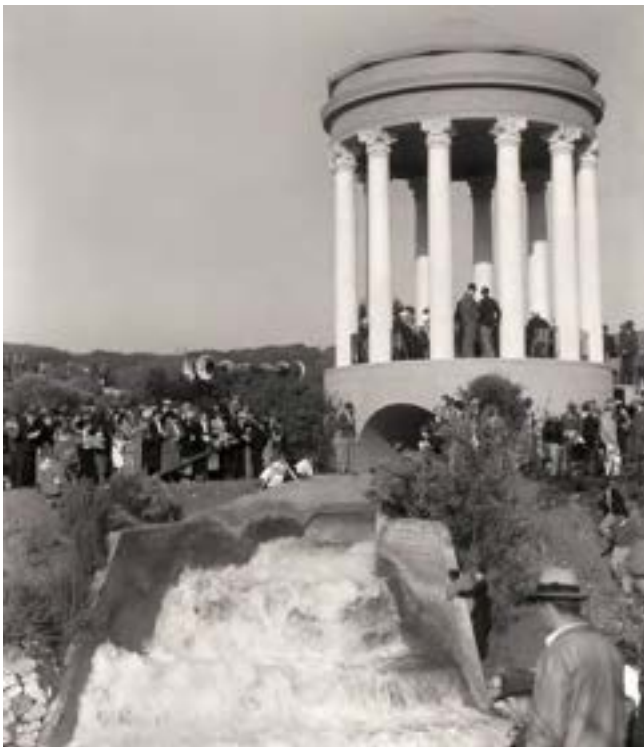
Figure 53. October 1934 celebration at the Pulgas Water Temple of the delivery of the first water from the Hetch Hetchy Reservoir reaching the San Francisco Peninsula (SF-PUC).
